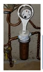
**WHOLE HOUSE SEDIMENT FILTER** (located below meter in photo to left): A budget friendly unit that most homes would benefit from as it physically removes particulates from the water before entering your home's plumbing. Advantages: Inexpensive and easy to install for those with lots of sand, silt or dirt in their water. Disadvantages: Ineffective in removing chemicals, bad taste, odor or any other contaminants. Requires replace of parts.
