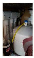
**REVERSE OSMOSIS SYTEM:** Reverse osmosis systems purify water through multiple stages usually including sediment filtration, ultraviolet light, deionization and the use of pre- and post-carbon filters in conjunction with the use of a reverse osmosis membrane. Advantages: Effective in removing a wide spectrum of contaminants to produce very pure water. Disadvantages: Very expensive. Takes out valuable minerals. Requires replacement of parts.
